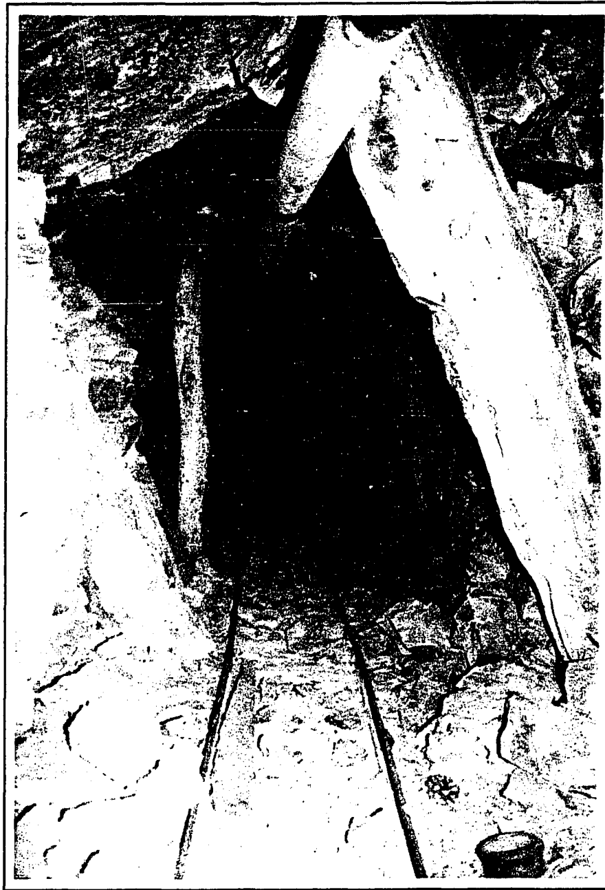
Figure 31. Adit at Locus 2, showing ventilation unit.
