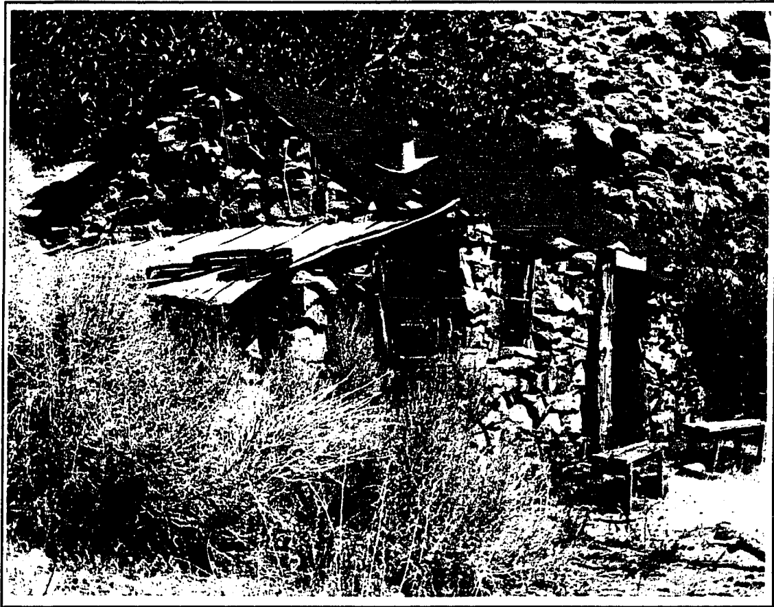
Figure 20. Stone masonry cabin with sheet metal roof, Locus 36.
