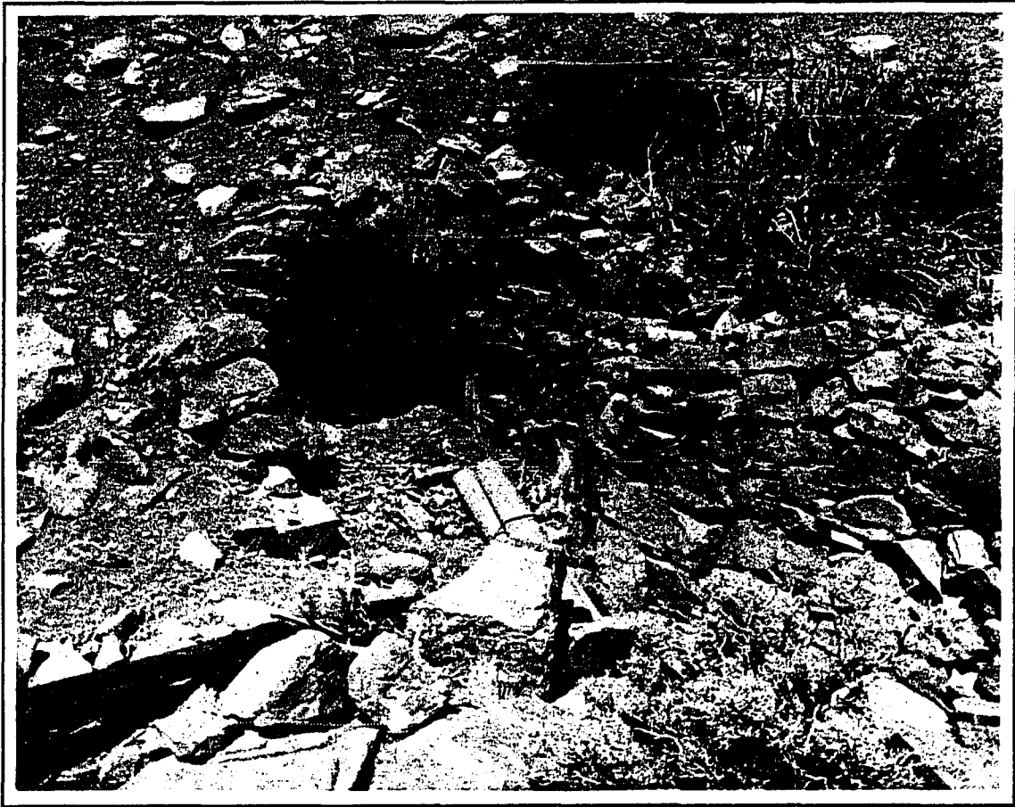
Figure 29. Rockwork retaining wall outside adit portal.
