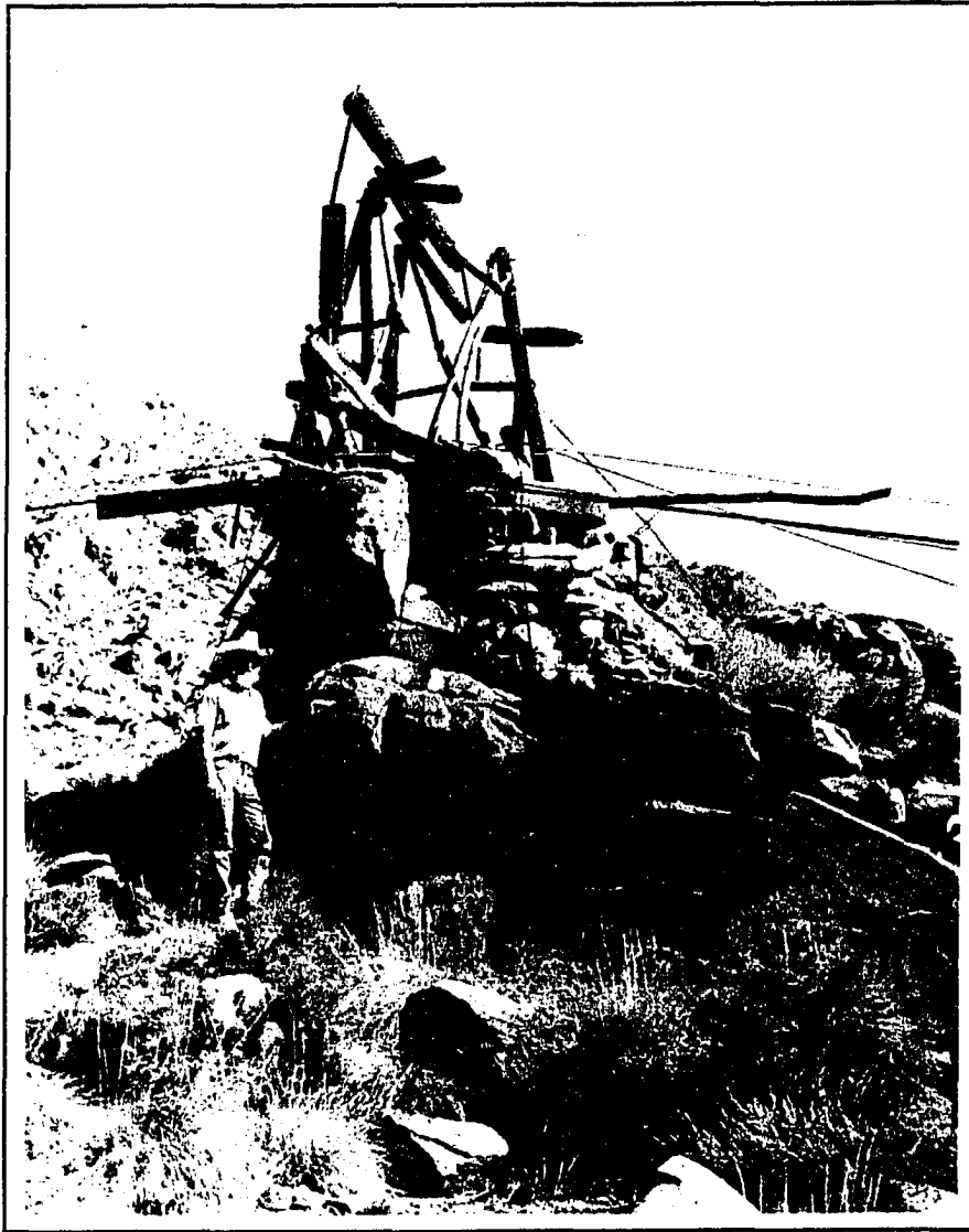
Figure 40. Intermediate station on aerial tram.
